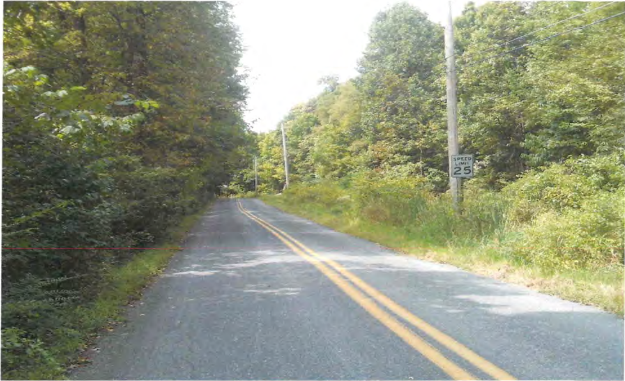
Photo O. Western view of Trail Road North in the vicinity of Wetlands 6 and 7.
