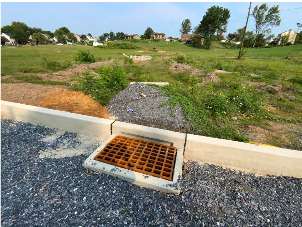
Figure 4: Inlet 29 has been installed (typ.) (9/13/2021)
