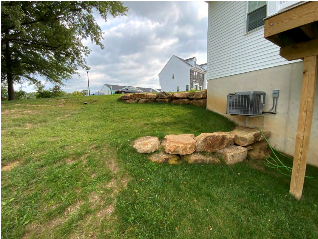
Figure 10: Three-foot retaining wall, installed as rock boulders, four-foot fence not installed (09/13/2021)
