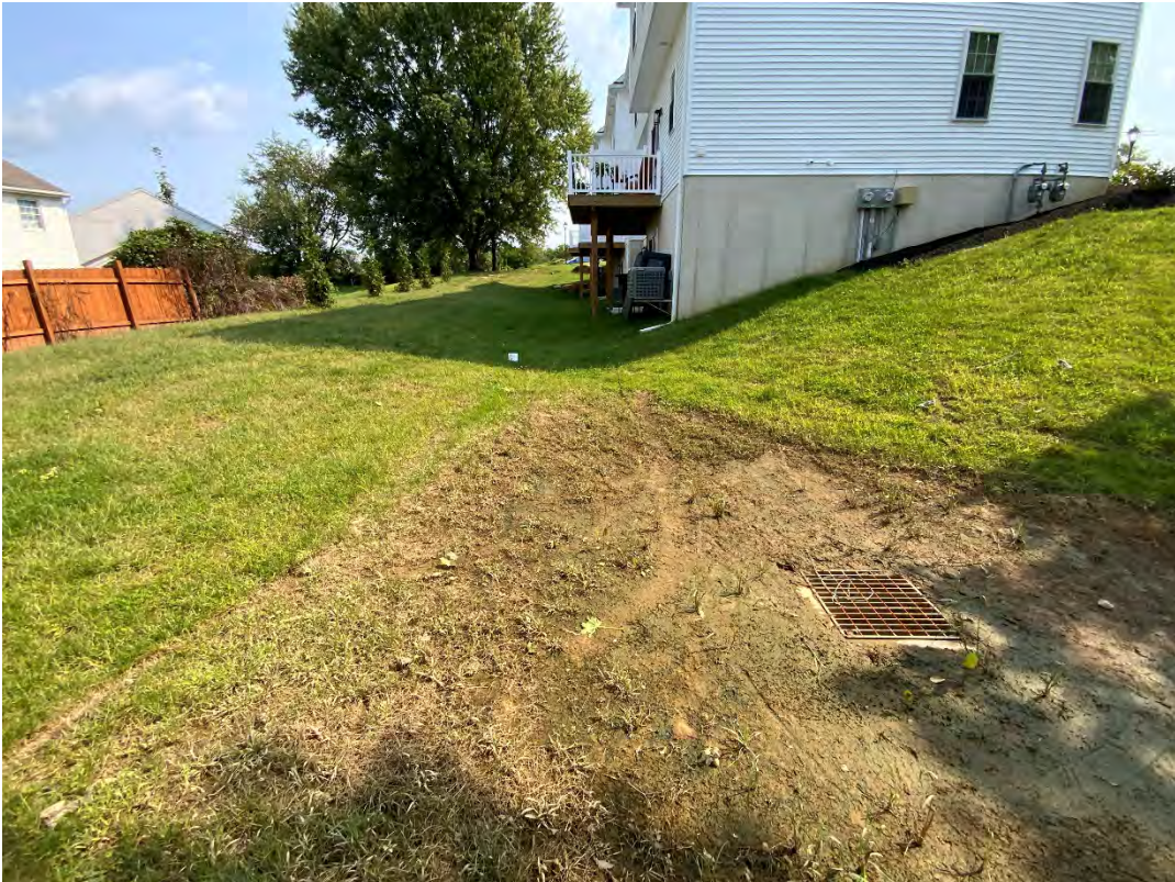
Figure 14: Swales were stabilized, except around I-A5 (typ.) (09/13/2021)
