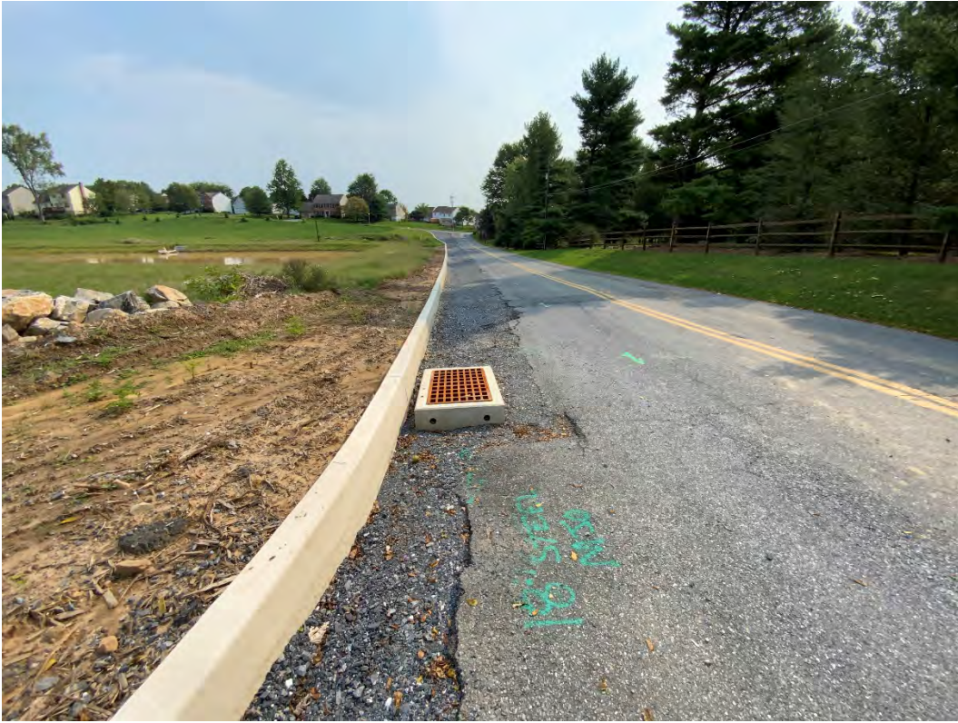
Figure 5: The pipe run from an existing inlet to IN-29 has been installed (typ.) (9/13/2021)
