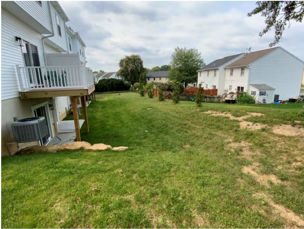
Figure 11: Gap in landscape screen where existing trees were removed (typ.) (09/13/2021)
