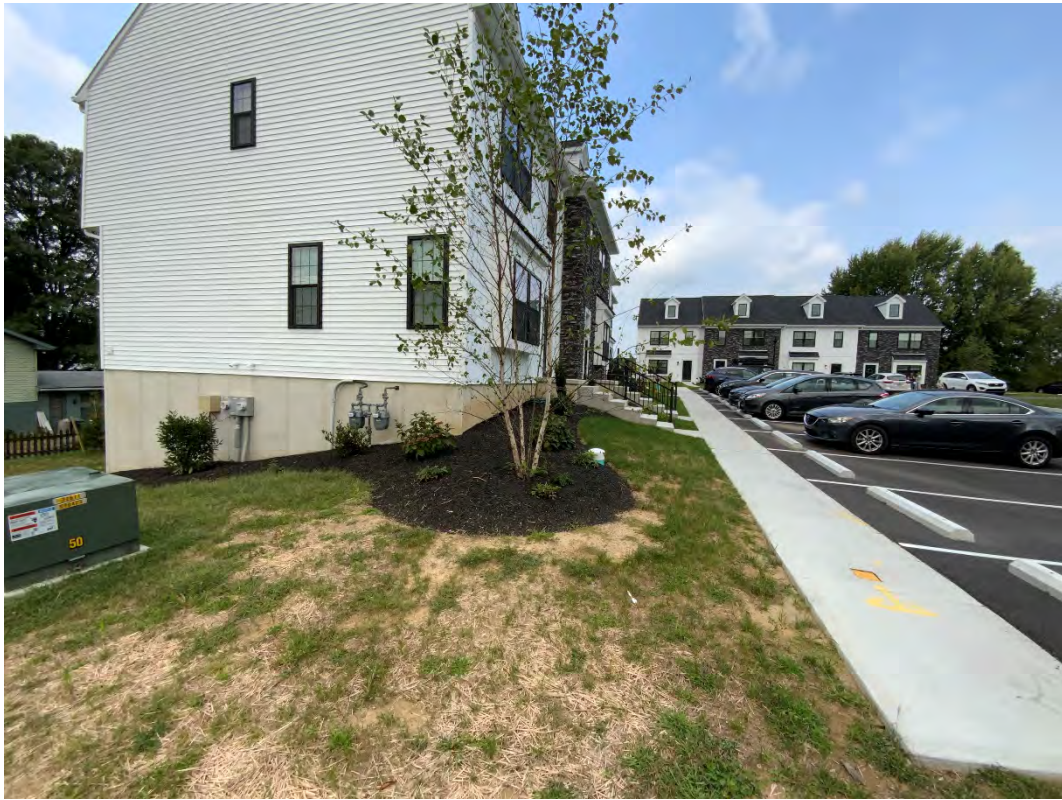
Figure 7: Concrete sidewalk and curb stops (typ.) (09/13/2021)
