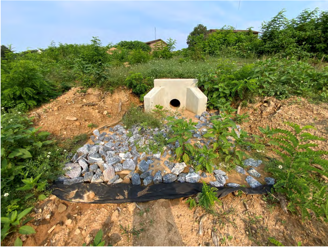
Figure 7: EW-12 has been installed (9/13/2021)
