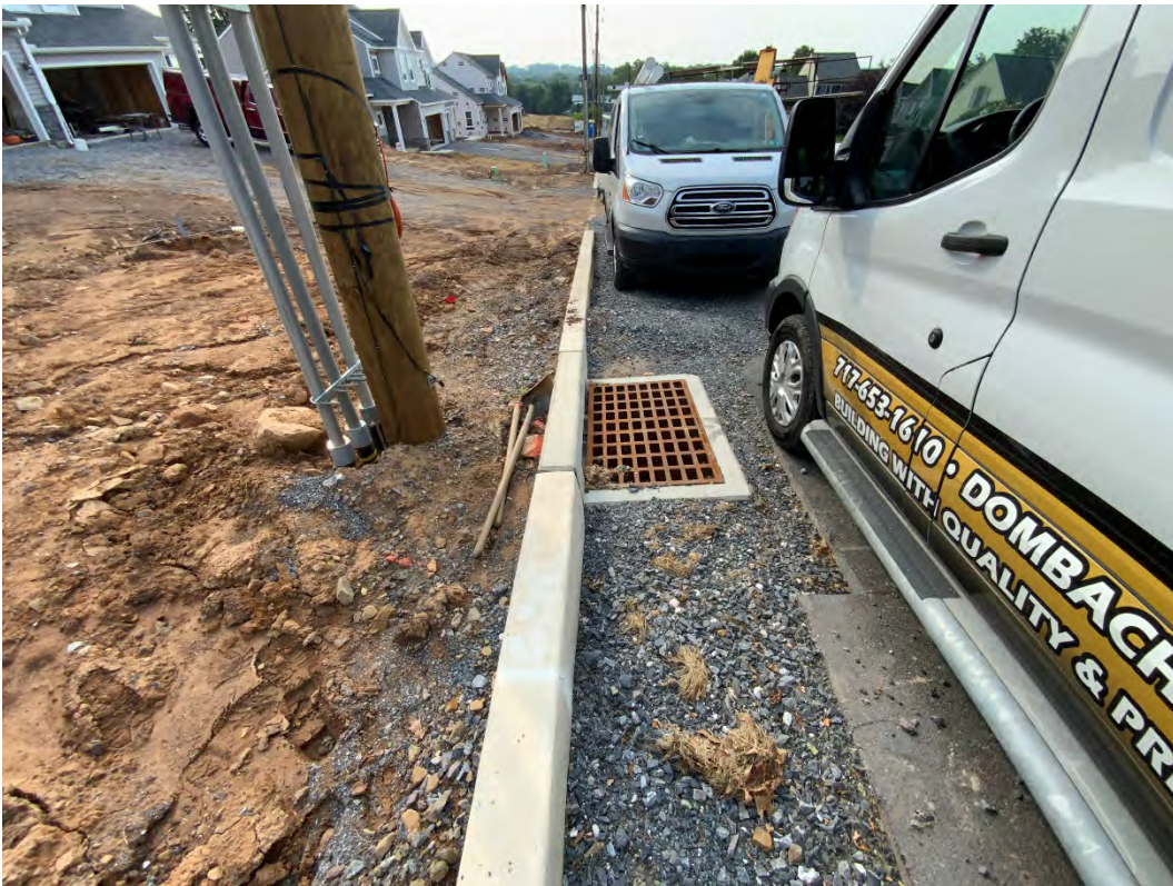
Figure 8: IN-13 has been installed (9/13/2021)
