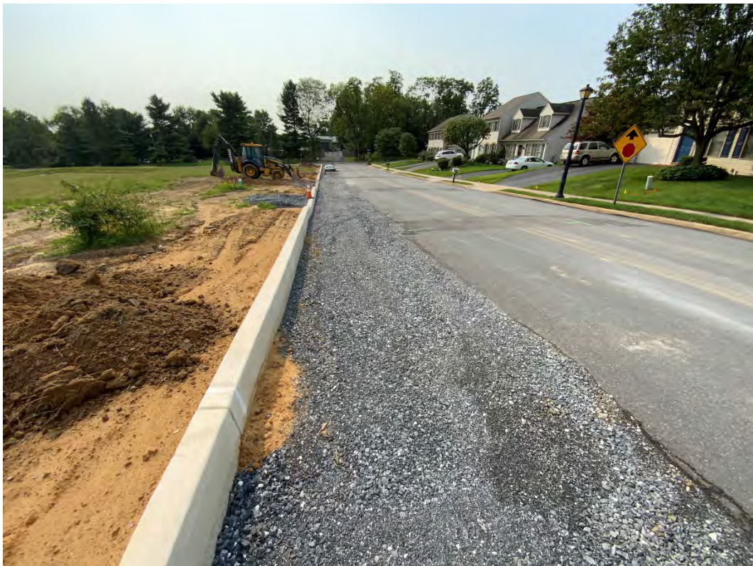
Figure 2: Vertical curbing and roadway subbase have been installed along Radio Road (typ.) (9/13/2021)
