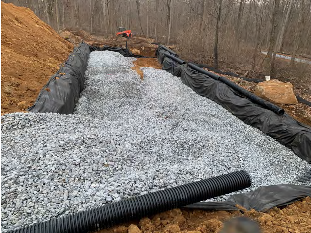
Figure 1: Infiltration Bed # 1 has been installed (photo taken 12/09/2021)
