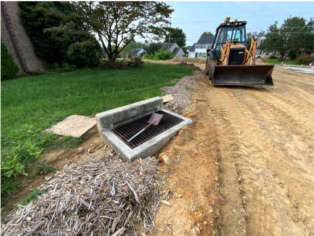
Figure 10: IN-17 has been installed (9/13/2021)
