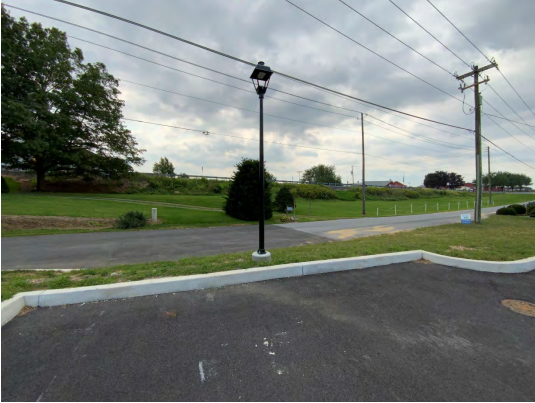
Figure 13: Lighting installed, different location than plans (typ.) (09/13/2021)
