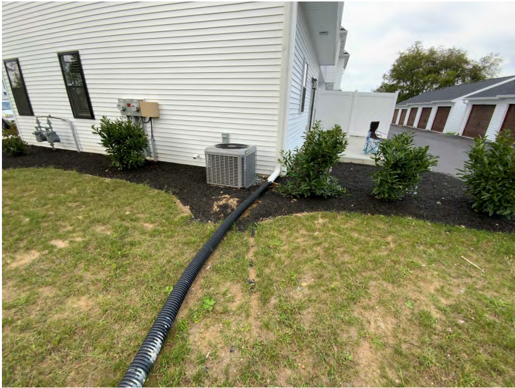
Figure 3: Downspout from eastern townhome not directed to Infiltration Bed #3 (09/13/2021)
