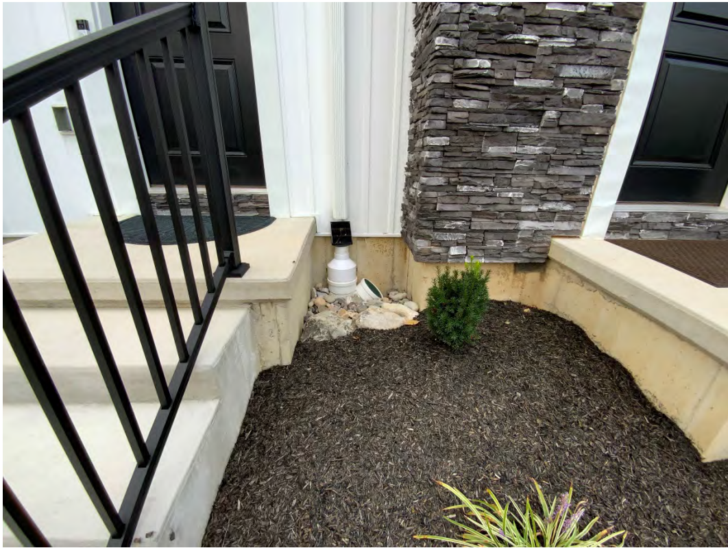
Figure 1: Downspouts were installed (typ.) (09/13/2021)
