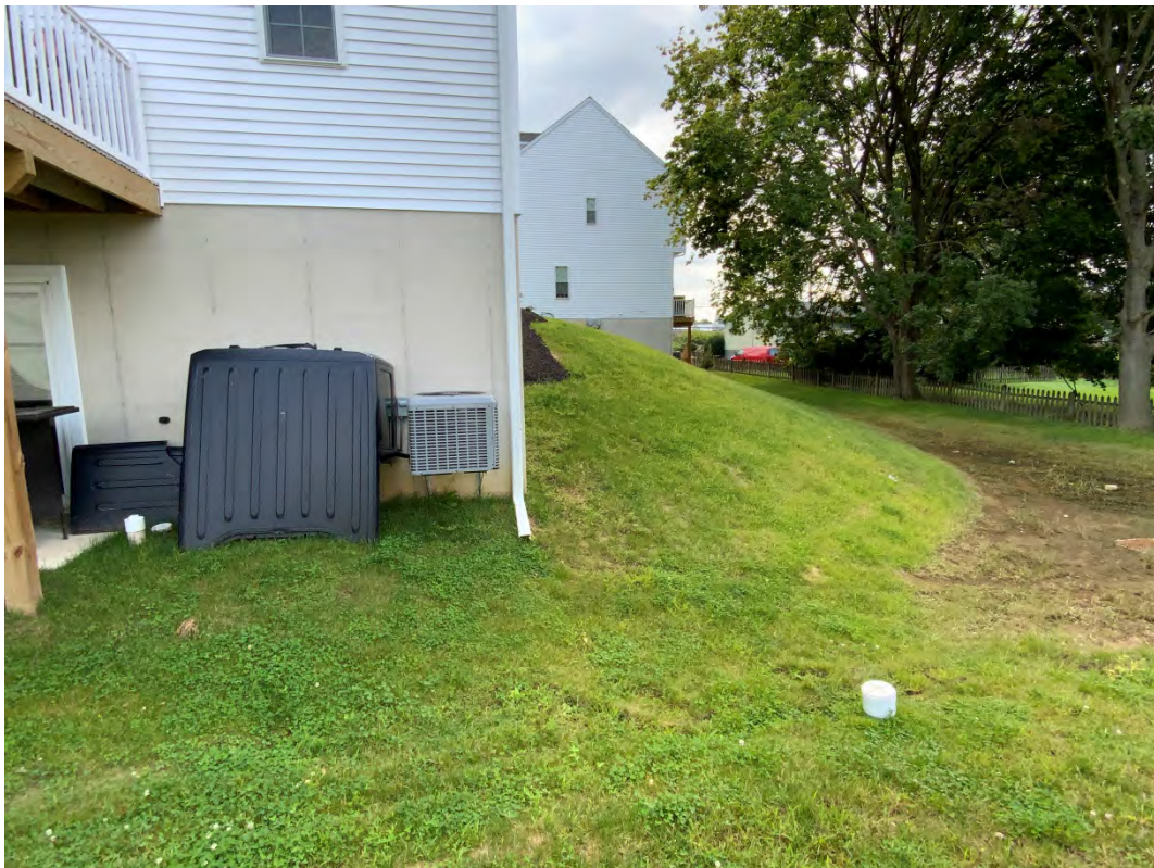
Figure 2: Downspouts discharging to grade without concrete splash blocks (typ.) (09/13/2021)
