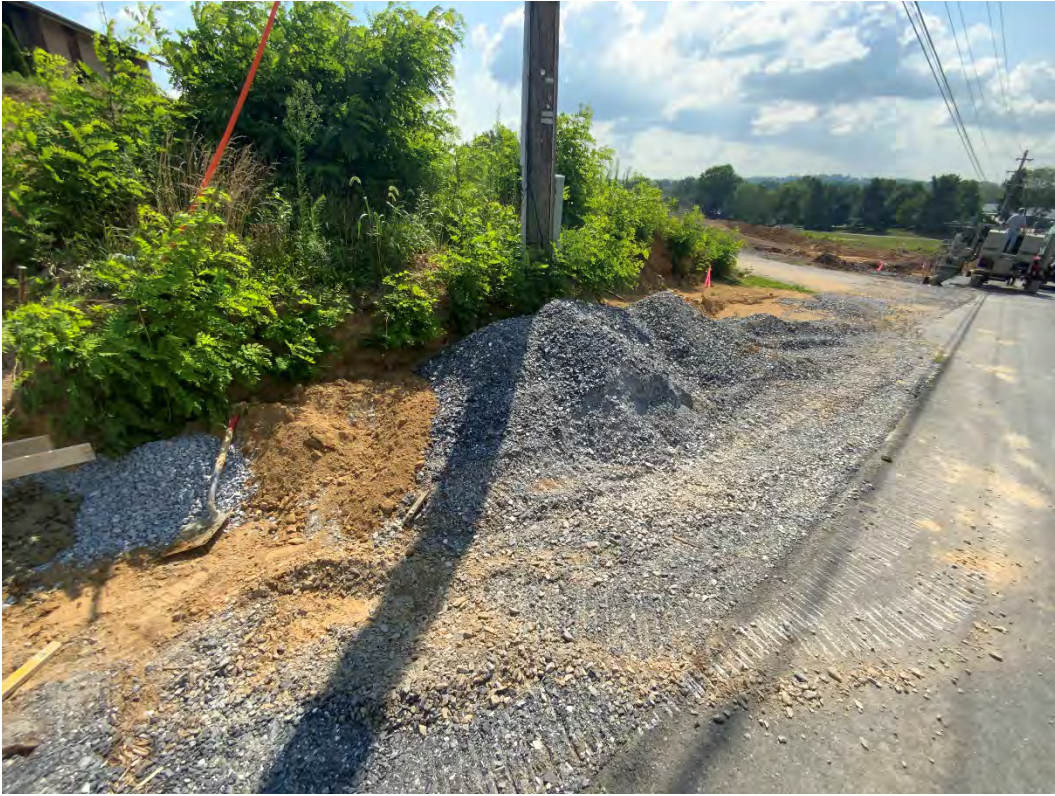
Figure 3: Portion of Radio Road where vertical curbing has not yet been installed (typ.) (9/13/2021)
