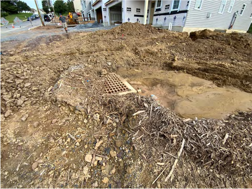
Figure 9: IN-18 has been installed (9/13/2021)
