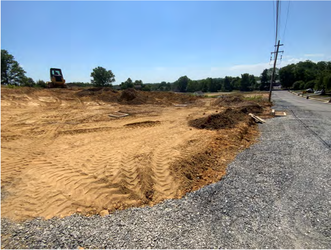
Figure 11: IN-19 and IN-20 have been installed (6/30/2021)
