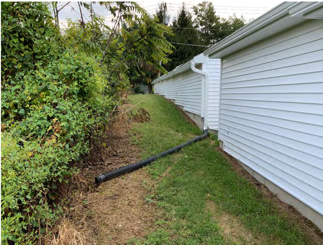
Figure 4: Downspouts from rear of storage units not directed to Infiltration Bed #3, two foot retaining wall not installed (09/13/2021)
