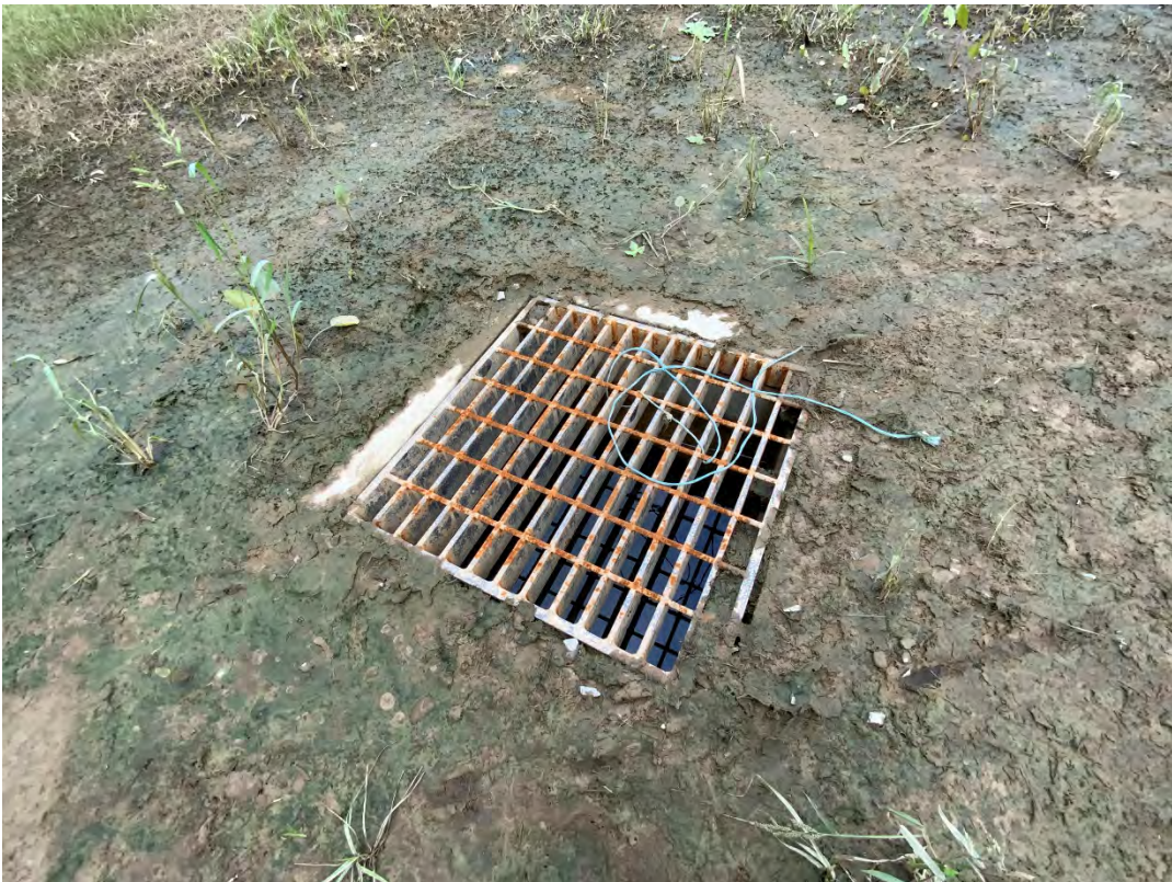
Figure 16: Standing water observed in I-A5 (09/13/2021)
