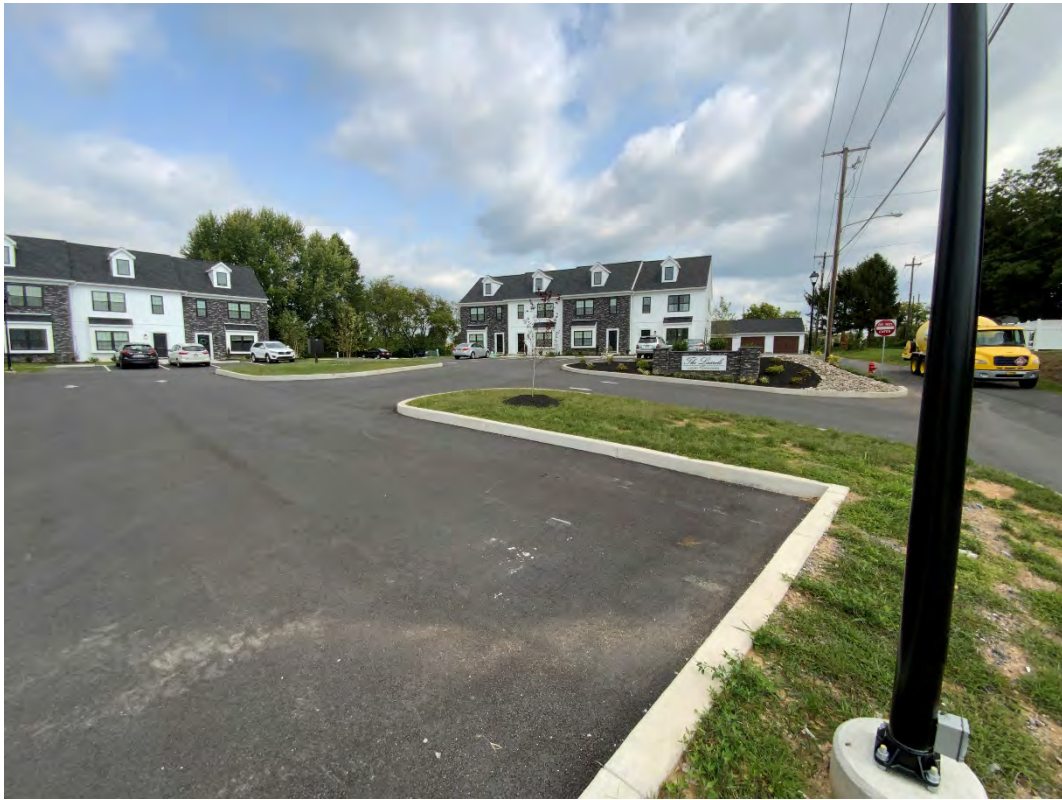
Figure 5: Asphalt wearing course installed in parking areas (typ.) (09/13/2021)
