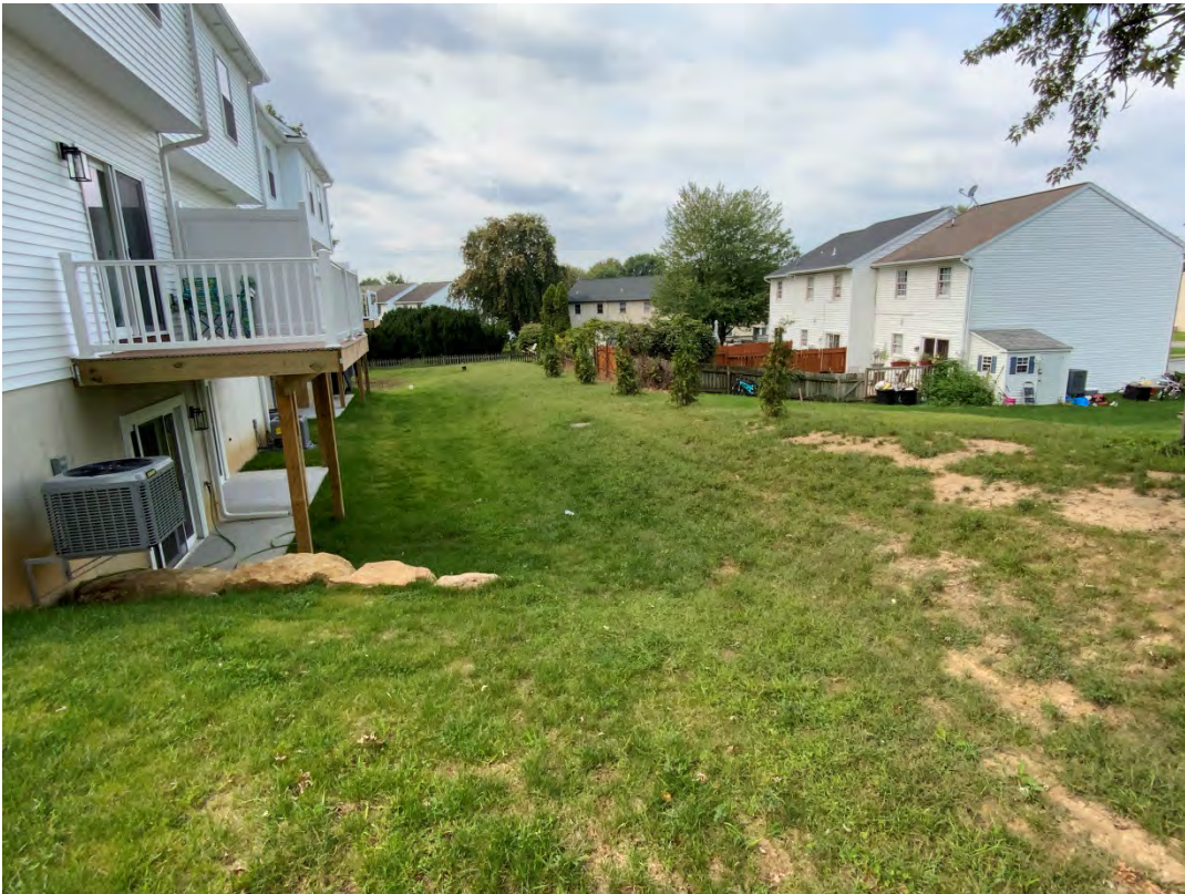
Figure 15: Portions of the site were stabilized, including some 3:1 slopes (typ.) (09/13/2021)
