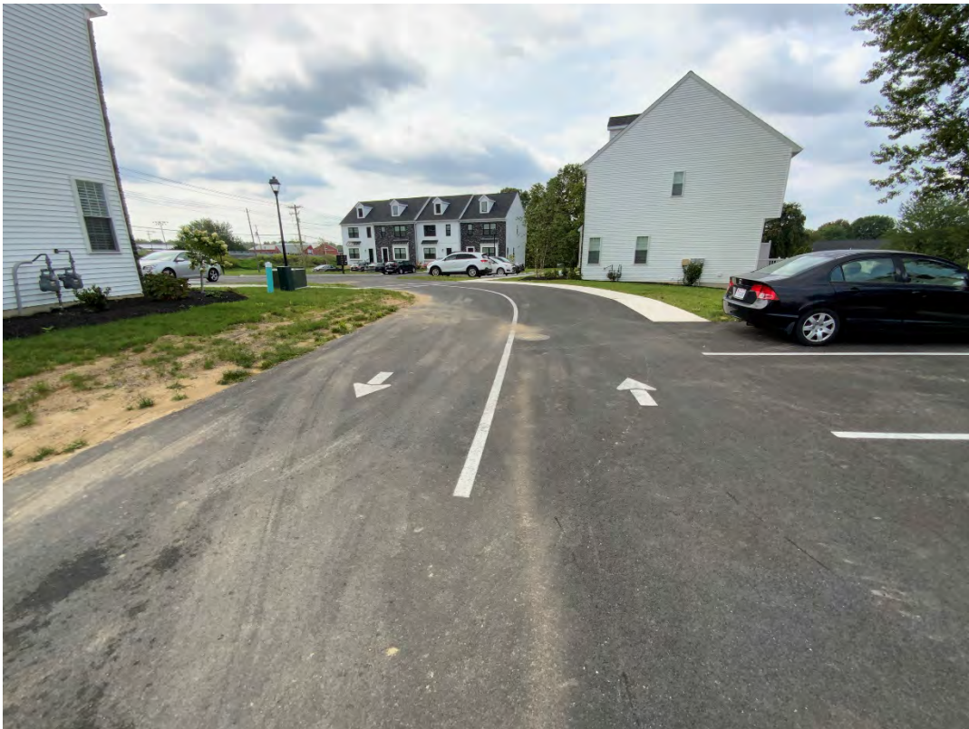
Figure 8: Paving markings were installed (typ.) (09/13/2021)
