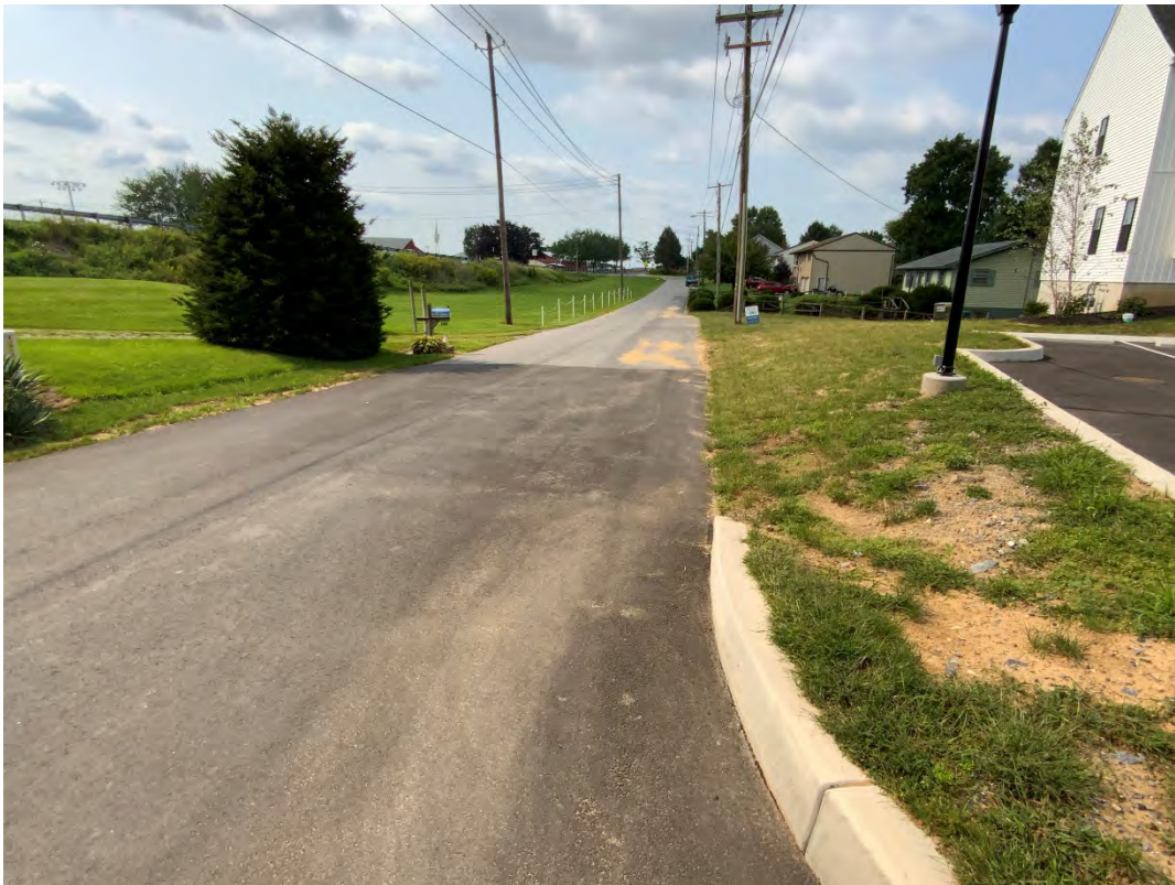
Figure 6: Asphalt wearing course installed for road widening (09/13/2021)
