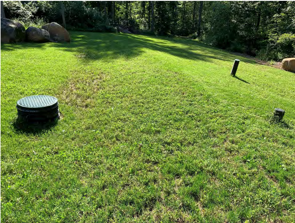
Figure 2: The cleanouts and Inlet 1 need to be cut flush with the finished grade (09/07/2021)
