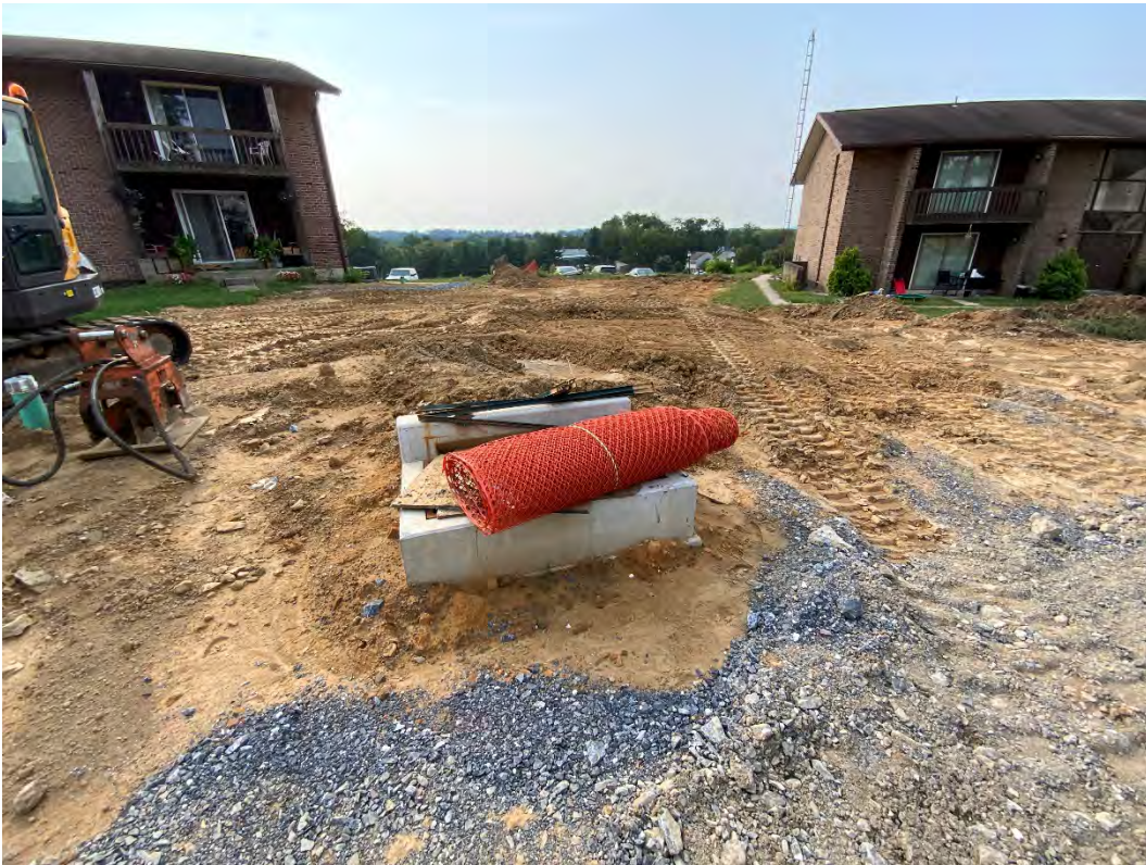
Figure 6: IN-9 has been installed (09/13/2021)
