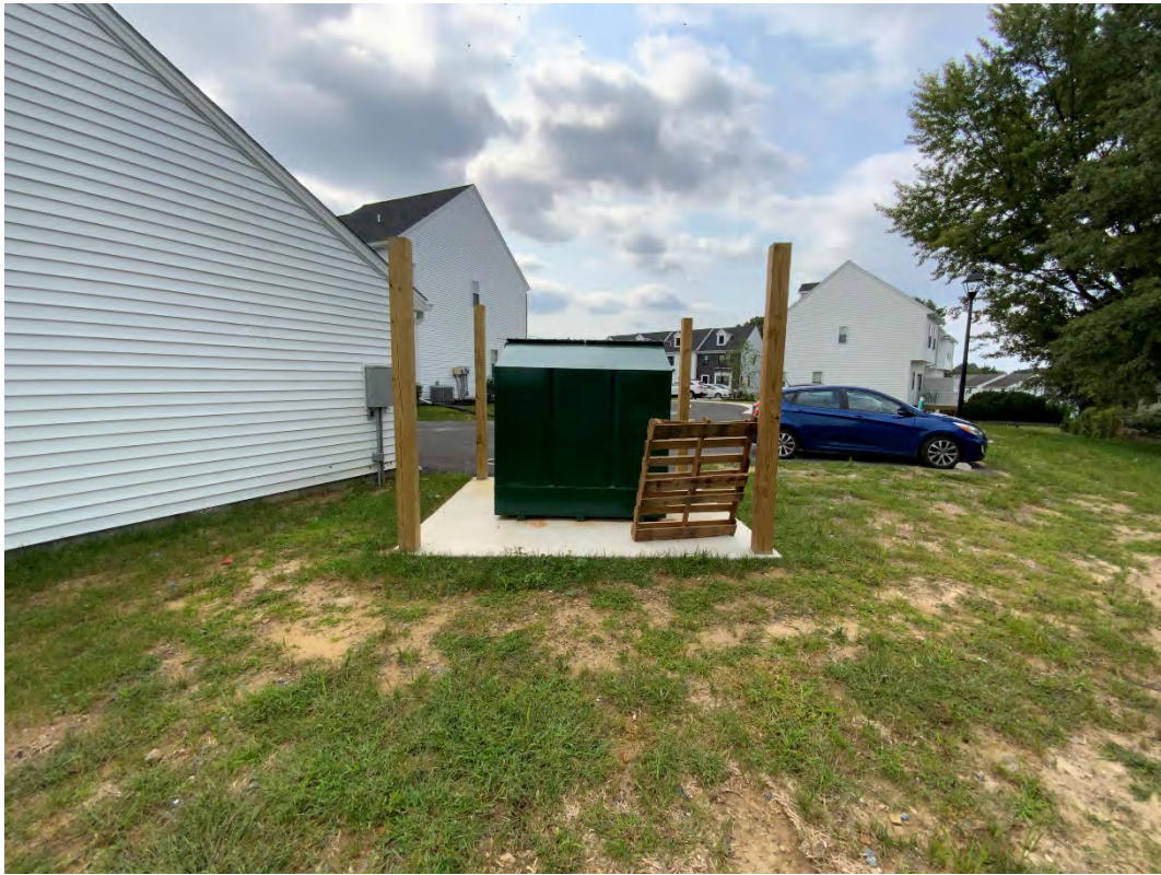
Figure 9: Dumpster enclosure was partially installed (09/13/2021)
